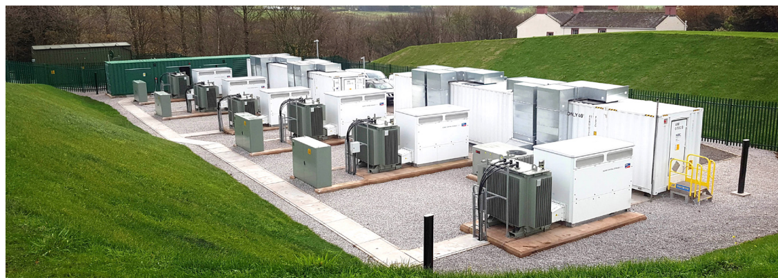
Cleator (c)2017 NEC Energy Solutions, Inc. - Image used with permission - 10MW project, located in Cumbria
